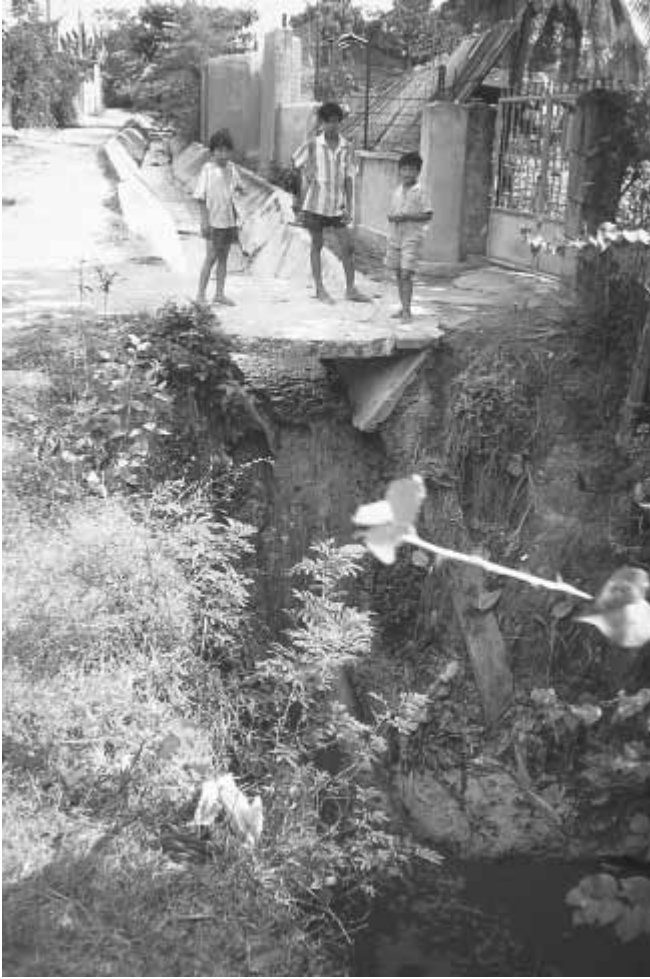
Figure 3.2 The wastewater canal for the Dona Bochang textile factory
